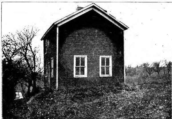
Fig. 71.—Shop (looking South).
